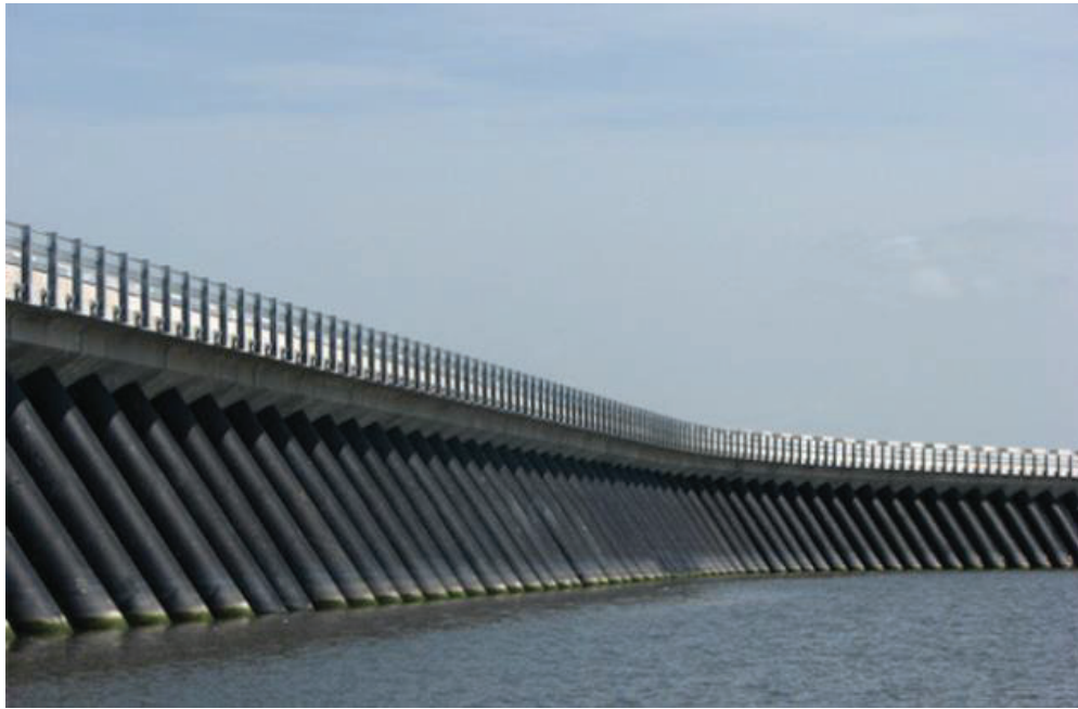
Example of a surge barrier wall in New Orleans, LA.
